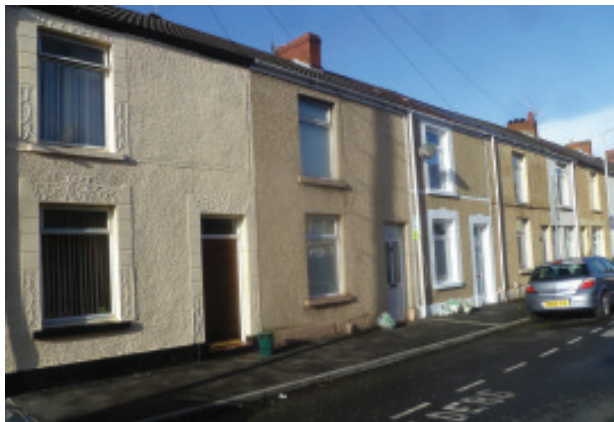
Typical Sandfields terraced Housing
