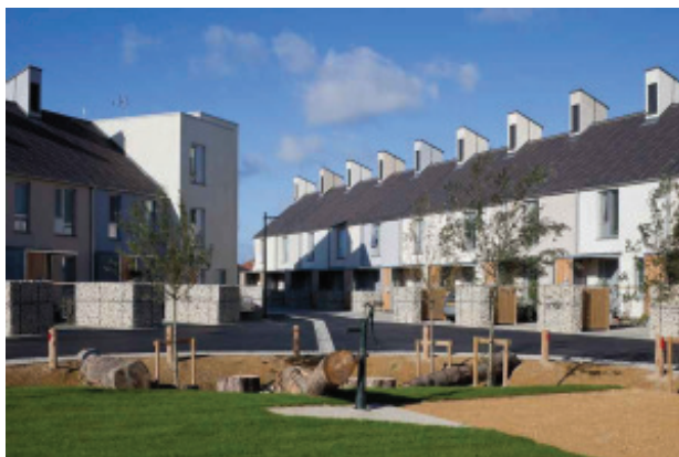
Swindon Triangle: contemporary terraces overlooking open space (Code for Sustainable Homes level 4)
